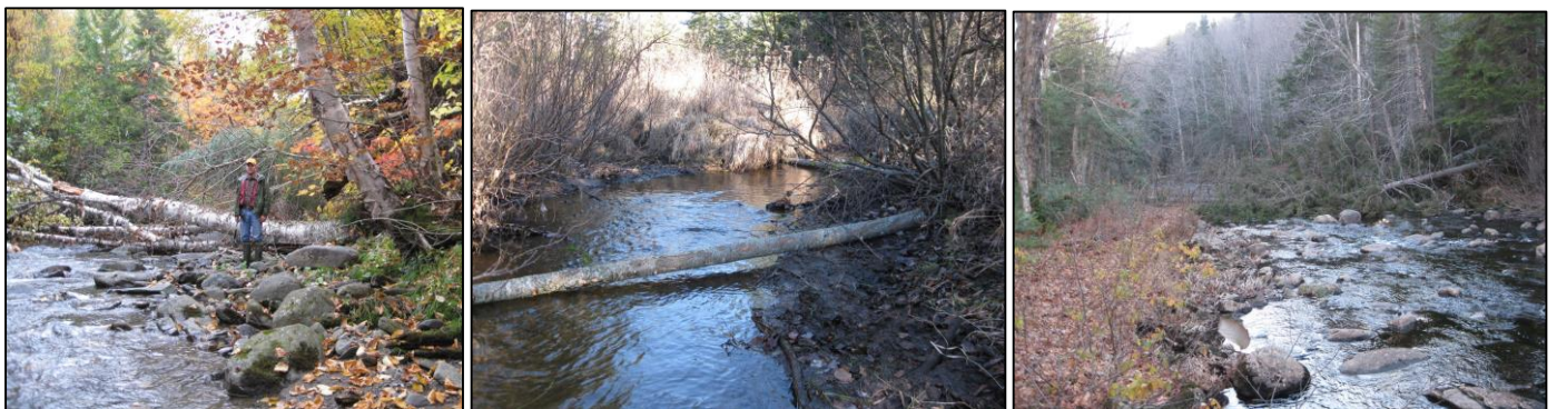
(L) Birch with root wad set into Intervale Bk, ME. (M & R) Two examples of “chop and drop” in the upper and middle portions of the East Branch Nulhegan River, VT. Fall 2012.
